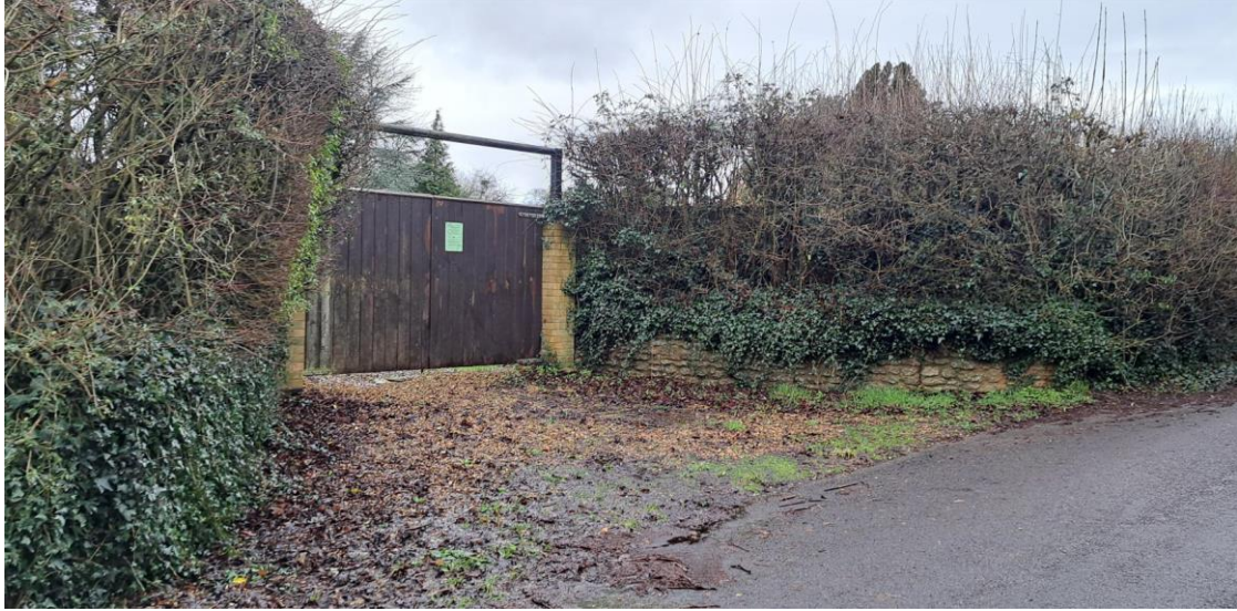
The existing site entrance
